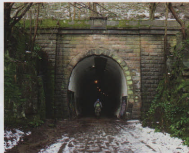
Below: Tunnel on the Upper Don Trail
